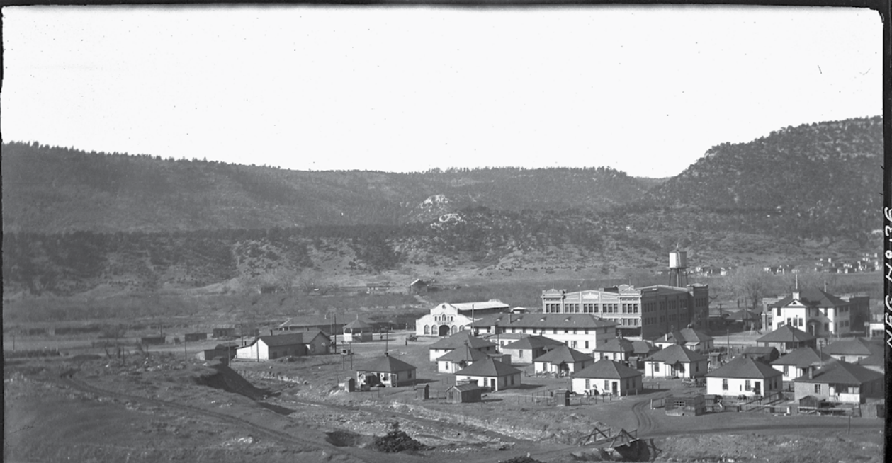
PHELPS DODGE STORE, WAREHOUSE & HOTEL, DAWSON, N.M. 11-20-20
